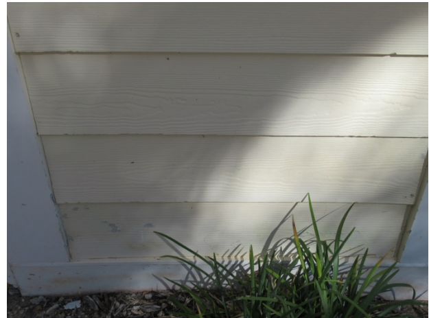
Finish deterioration at Heritage A pool house, note – budget for paint applications through operating budget
