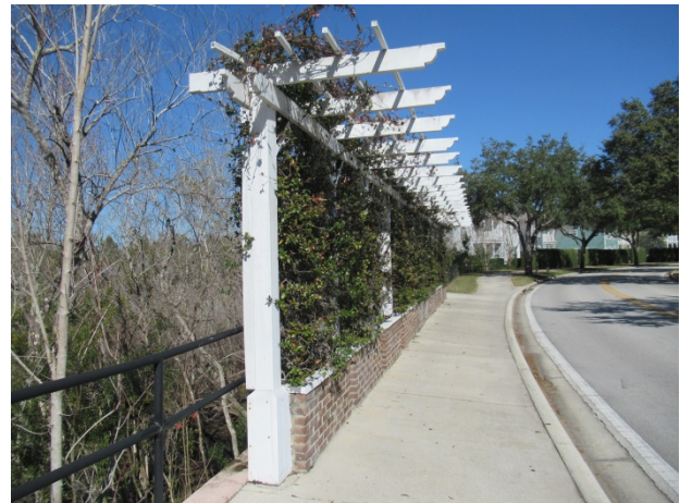
One of two trellises at Reunion Boulevard
