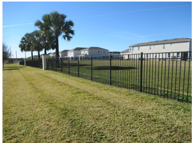
Perimeter fence at Encore phase
