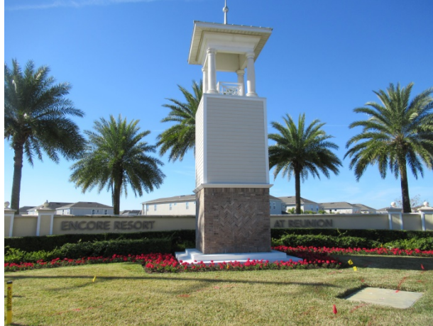
Entrance monument at Encore phase
