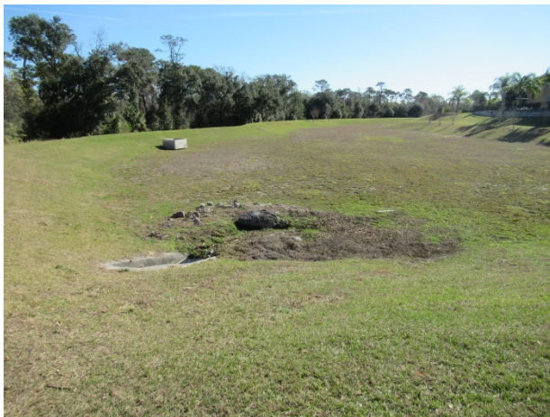
Storm water detention basin at Encore phase
