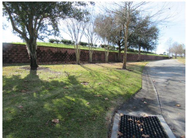
Retaining wall near The Terraces
