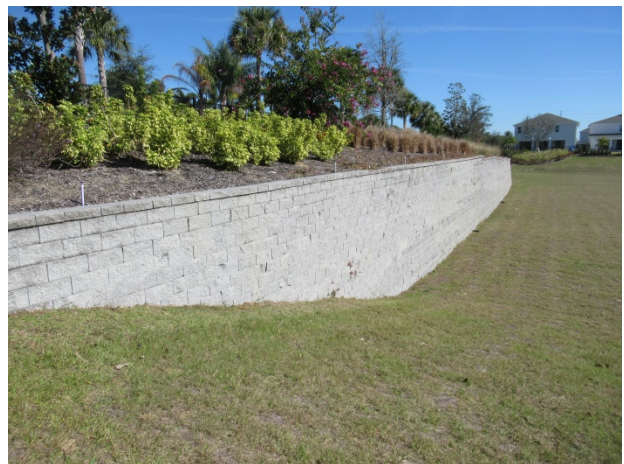
Retaining wall at Encore phase detention basin
