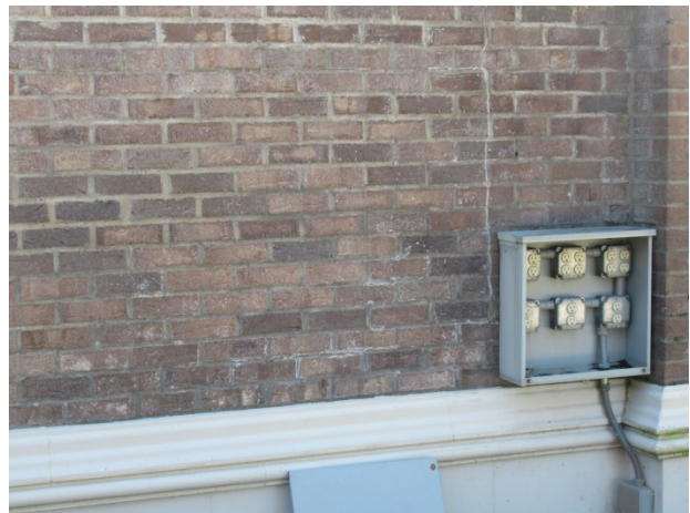
Minor efflorescence
