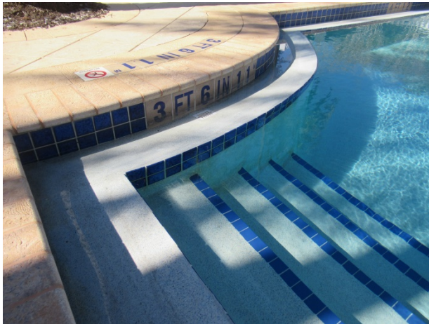
Finishes at Heritage A
