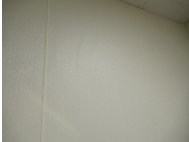
Plastic wall covering at kitchen
