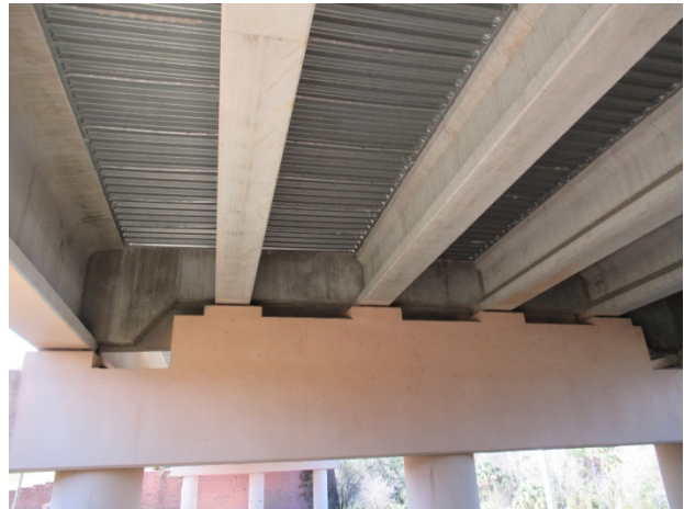
Gathering Drive bridge
