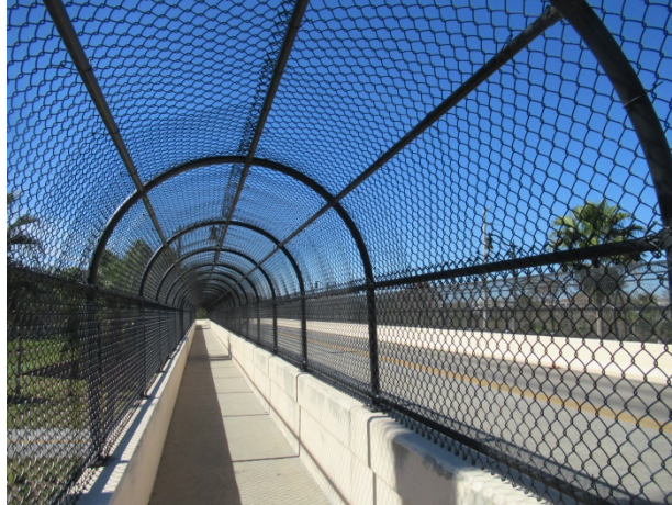
Fencing at Gathering Drive bridge
