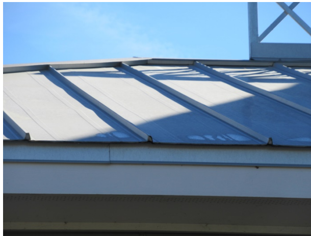
Standing seam metal roofing
