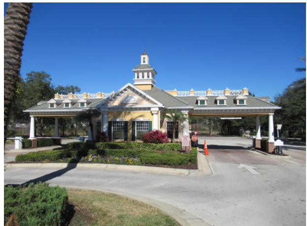
Main gate house
