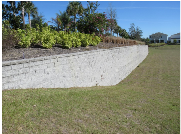
Retaining wall at Encore phase detention basin
