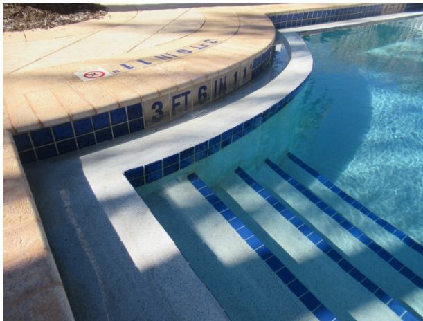
Finishes at Heritage A
