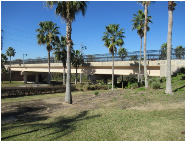
Gathering Drive bridge
