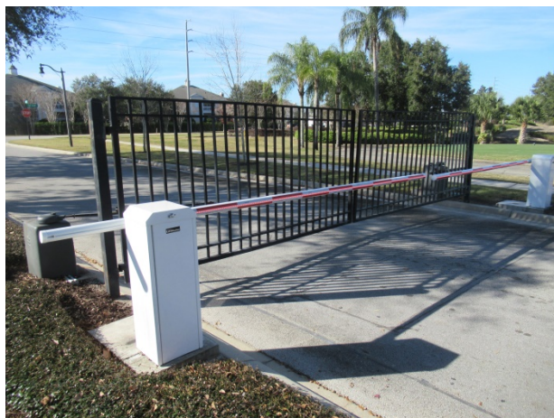
Gate arms and bi-parting gates
