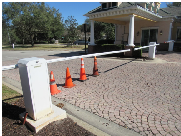
Gate arms and operators
