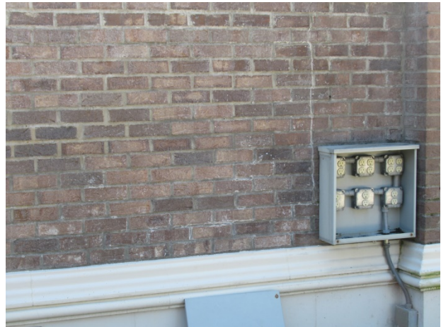
Minor efflorescence
