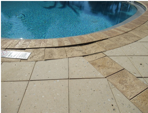
Isolated settlement at Homestead
