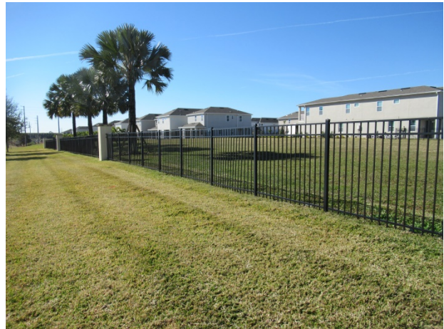
Perimeter fence at Encore phase
