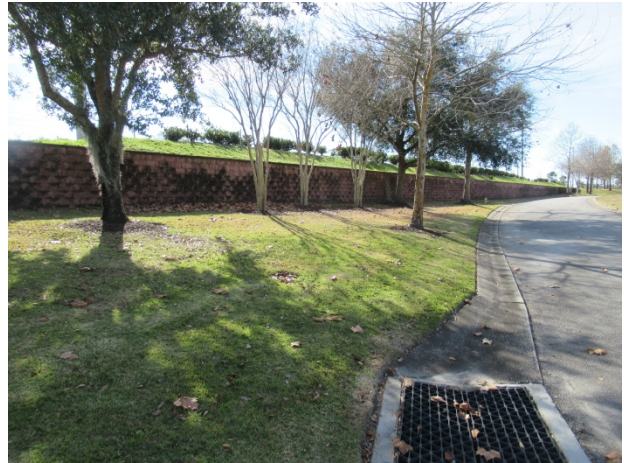
Retaining wall near The Terraces
