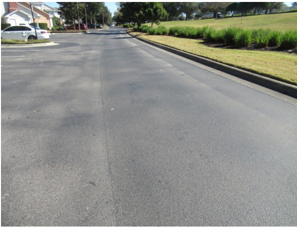
Asphalt pavement street at Heritage Crossing
