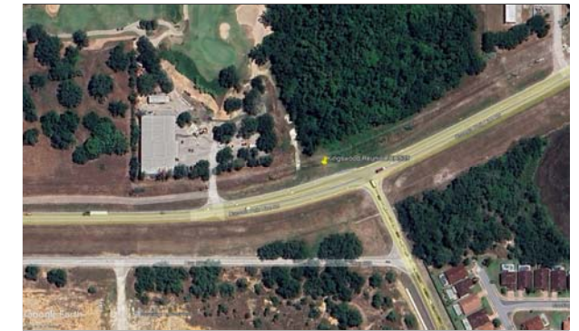
VICINITY MAP NEAR 7385 OSCEOLA POLK LINE ROAD, KISSIMMEE, FL 34747 (NOT TO SCALE)
