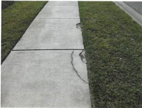
Concrete sidewalk cracks and damage
