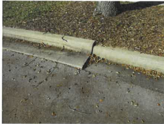
Settlement at curb and gutter
