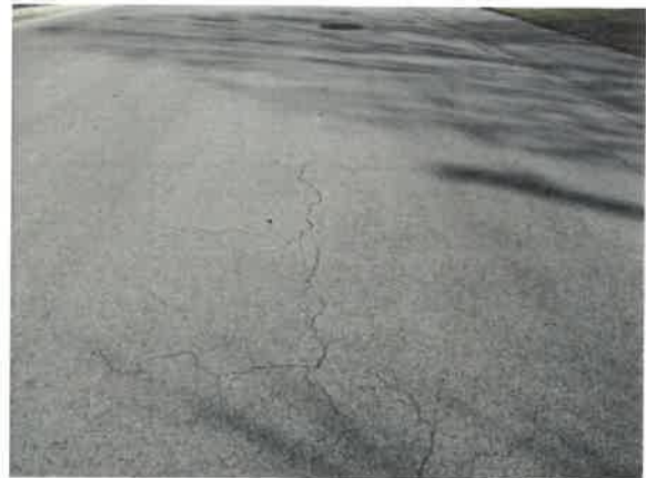
Minor cracks at Excitement Drive
