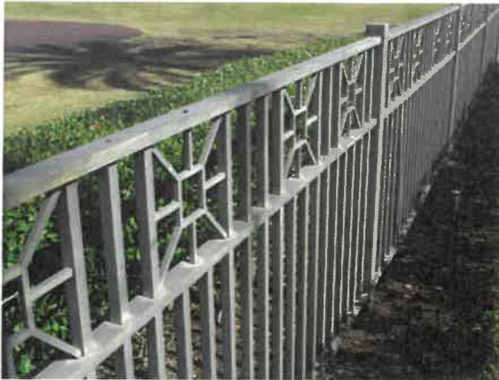
Typical aluminum fence, note fade
