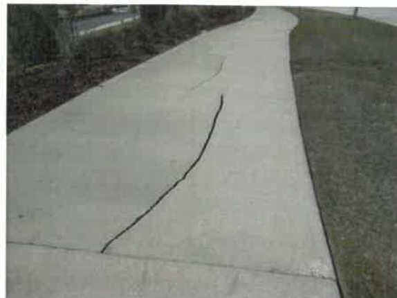
Sidewalk cracks near Tradition Boulevard gate house
