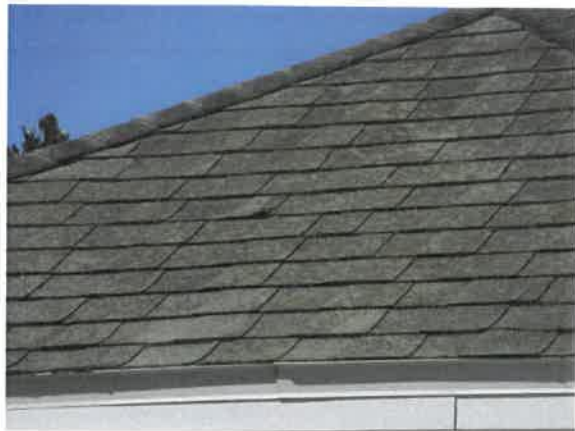
Shingle deterioration at Heritage B pool house
