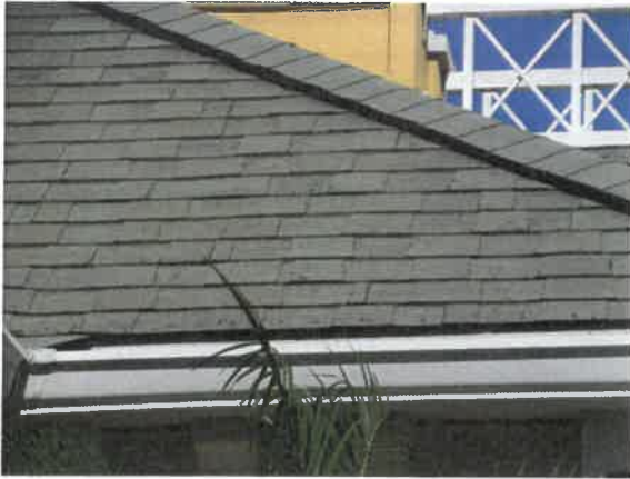
Granular loss at shingles at main gate house
