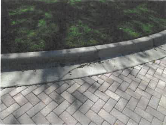
Minor concrete crack at curb and gutter
