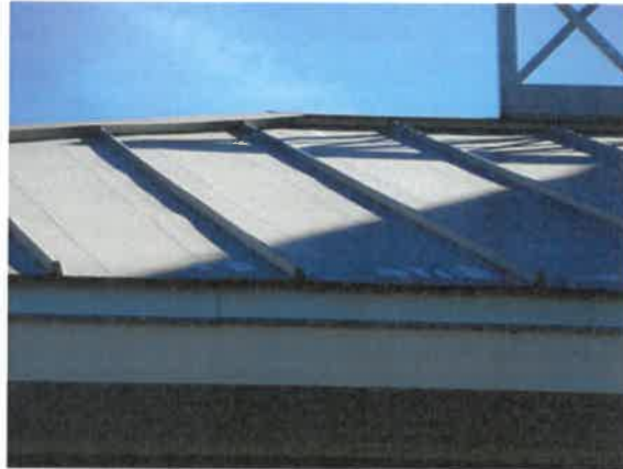
Standing seam metal roofing
