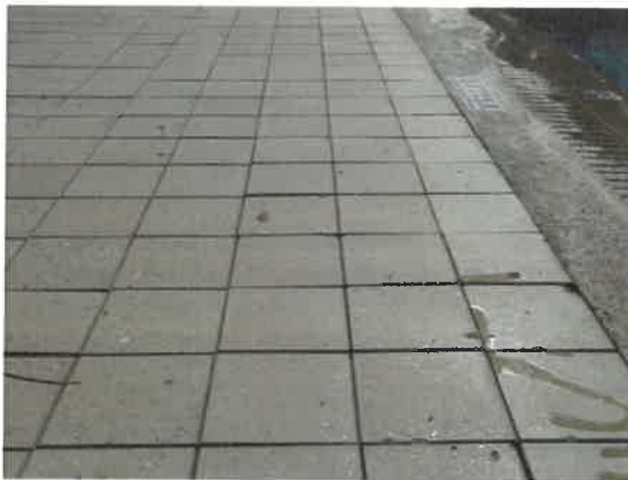
Spalls and minor settlement at Seven Eagles
