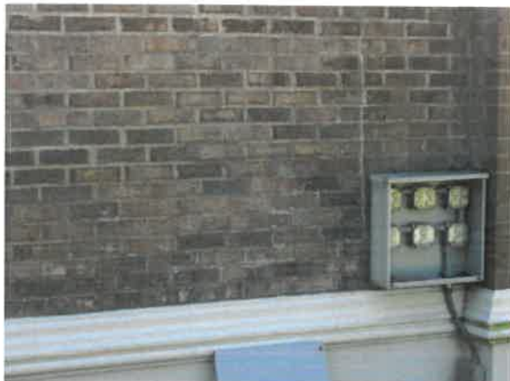
Minor efflorescence
