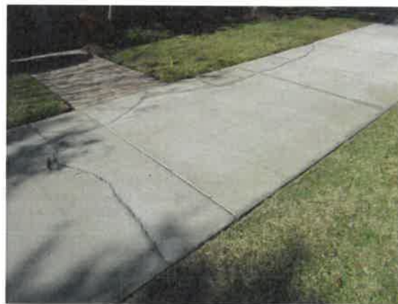
Multiple concrete sidewalk cracks near 1420 Reunion Boulevard
