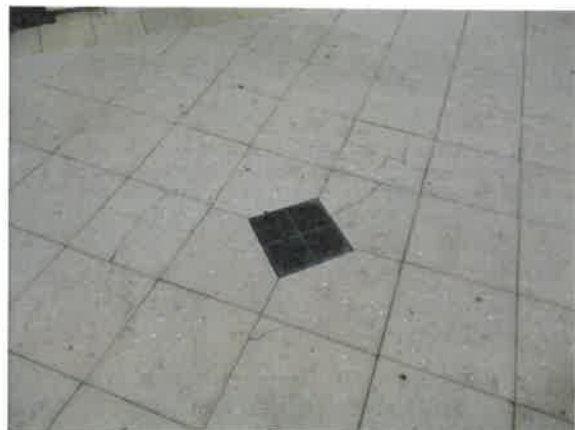
Cracked pavers at Carriage Point
